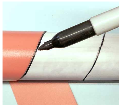
Figure 4: Drawing the guideline for accurately applying the copper tape
